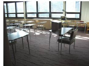
Priority 4 Example Replace worn interior finishes
