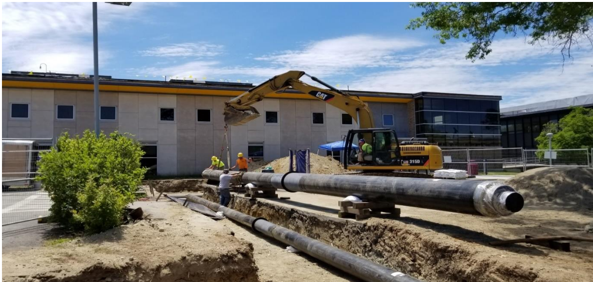
Alger Hall New Steam/Condensate Run
