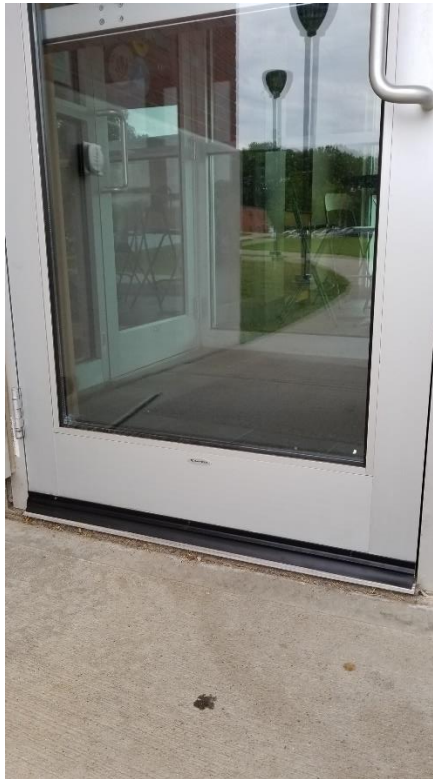
Building 5 New Door Sweep
